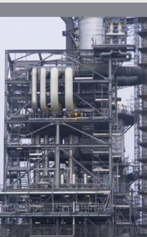
On-site job – refinery.
